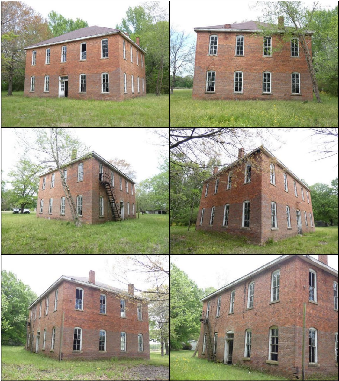
Figures 1 – 6 Overall exterior views.
