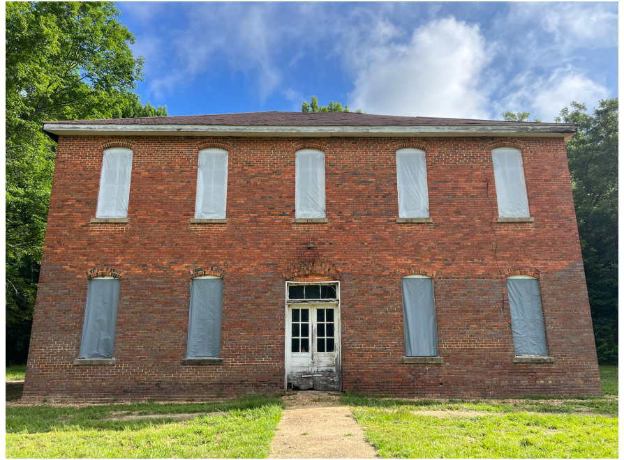
1B.2 South façade – facing north
