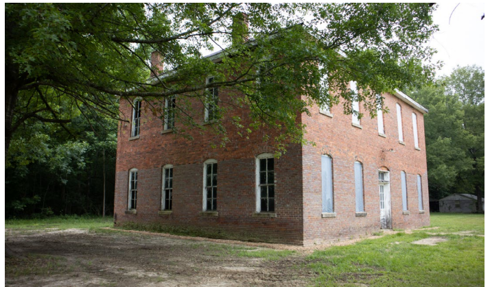
1A.4 Looking Northeast
