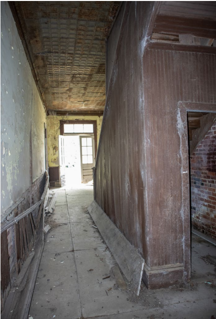
1C.13 Hallway – Looking West toward the primary entrance
