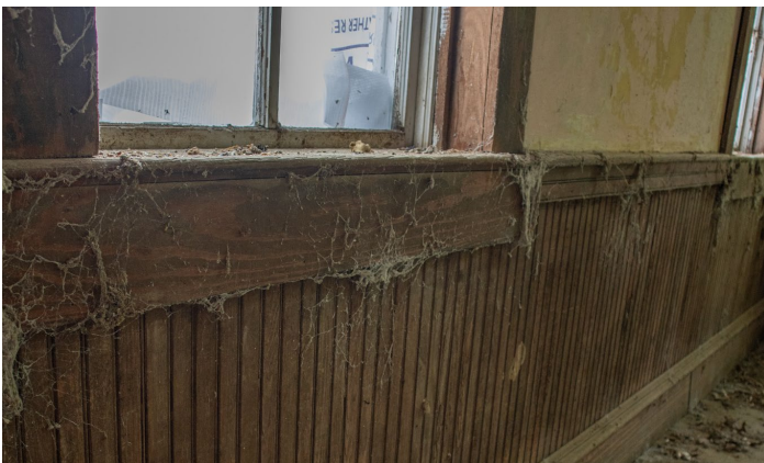
1D.20 Room B – Detail of window apron and beadboard wainscoting
