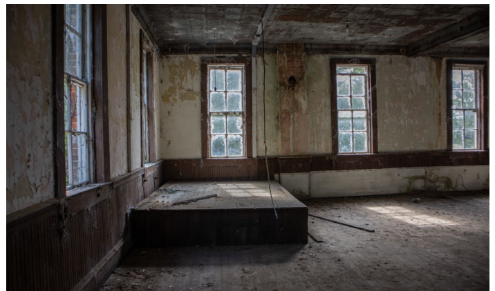
1D.6 Room A – Looking East
