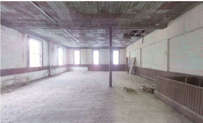
1D.8 Room A – Looking South
