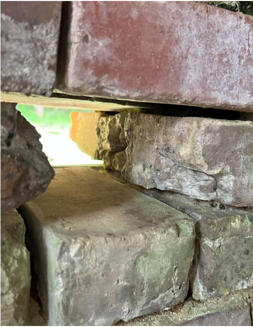
IC.41 Room B – Opening in northernmost masonry wall
