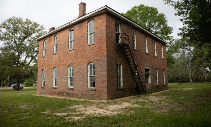
1A.1 Looking Southwest – In 2023 a French drain was installed around the perimeter of the building
