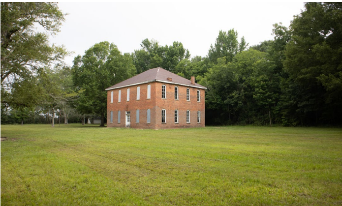
1A.3 Looking Northwest
