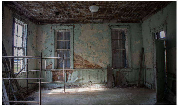
IC.20 Room A – Looking South
