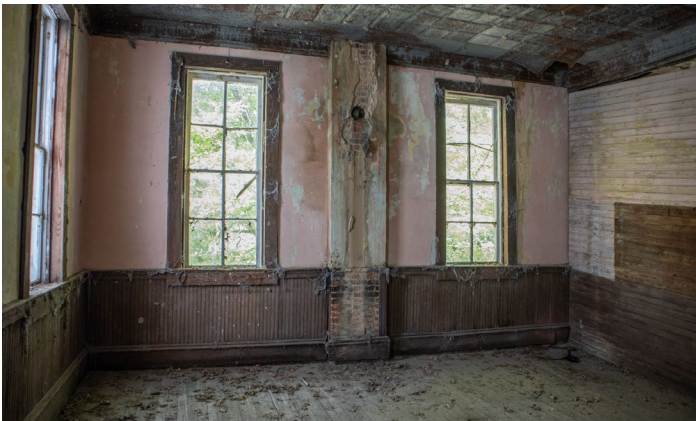
1D.18 Room B – Looking West - Notice chimney connection
