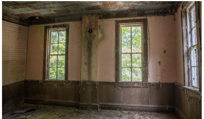
1D.25 Room C – Looking West - Notice chimney connection
