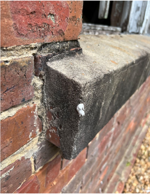
1B.24 East façade – Detail of lower story window concrete sill casing
