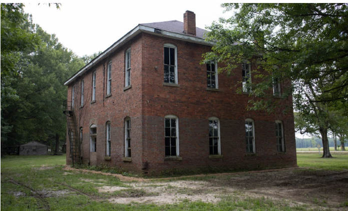
1A.5 Looking Southeast
