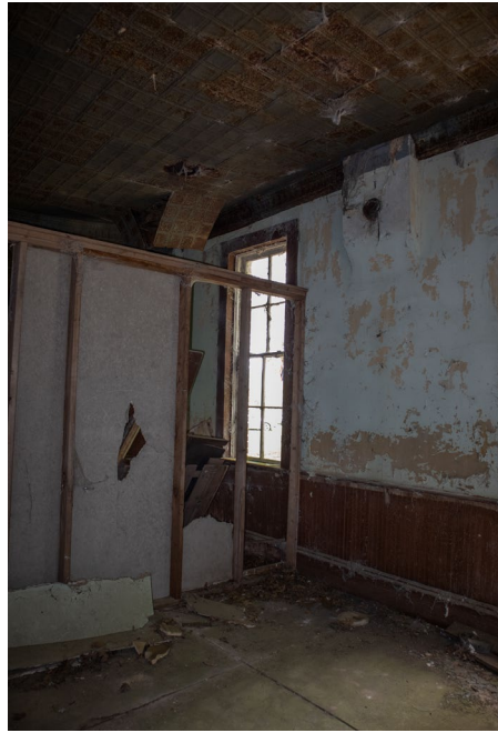
IC.46 Room B - Notice chimney connection
