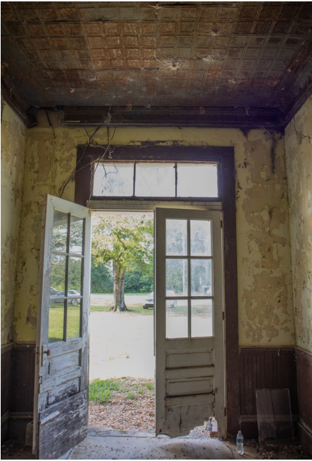
1C.1 Hallway - Primary entrance
