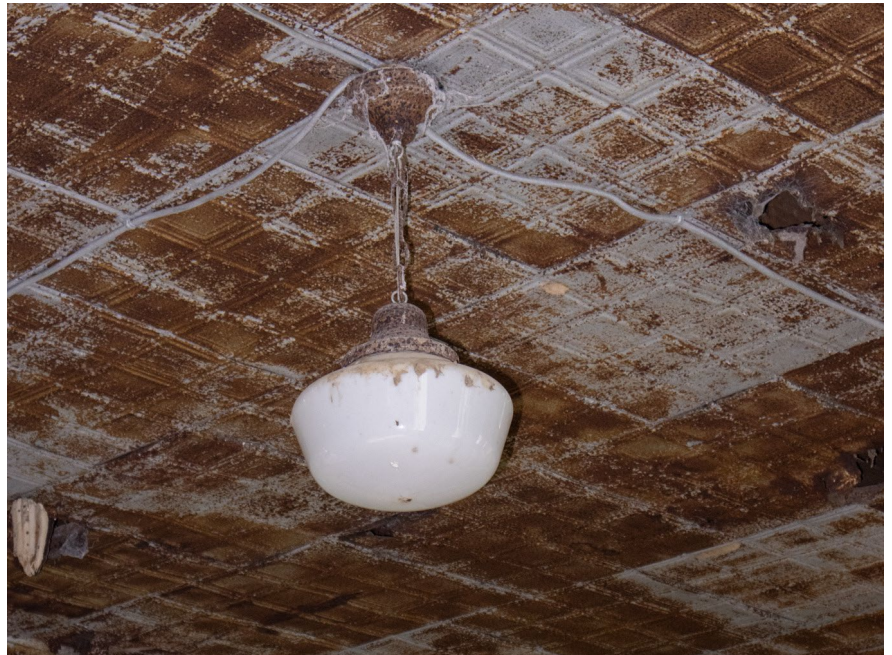
IC.34 Room A – detail of historic pendant lighting
