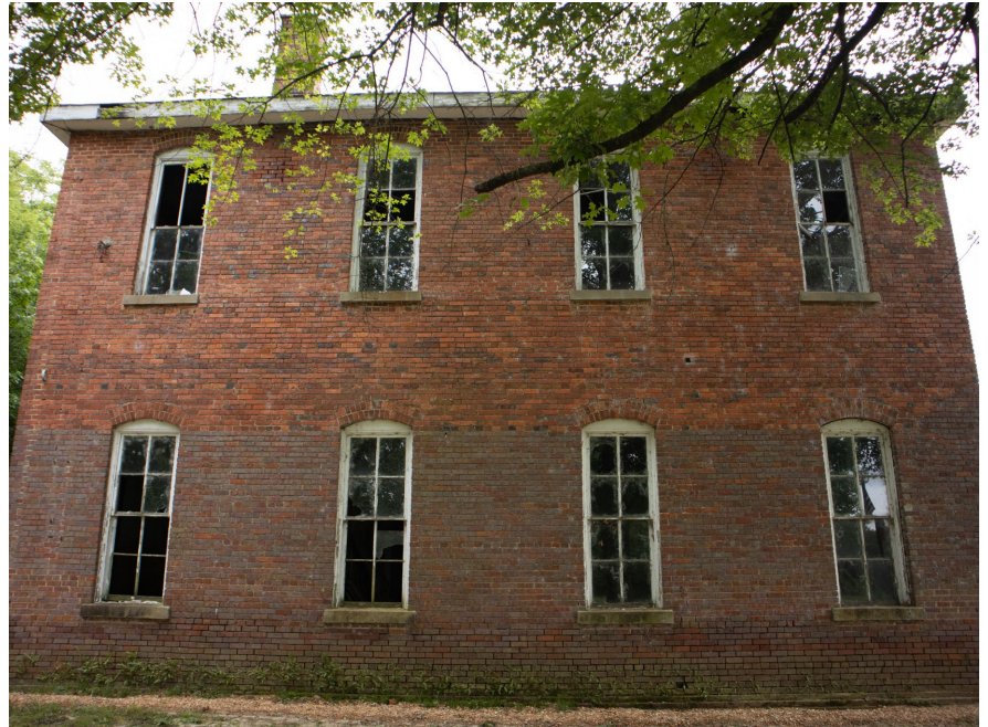
1B.9 West façade – facing east
