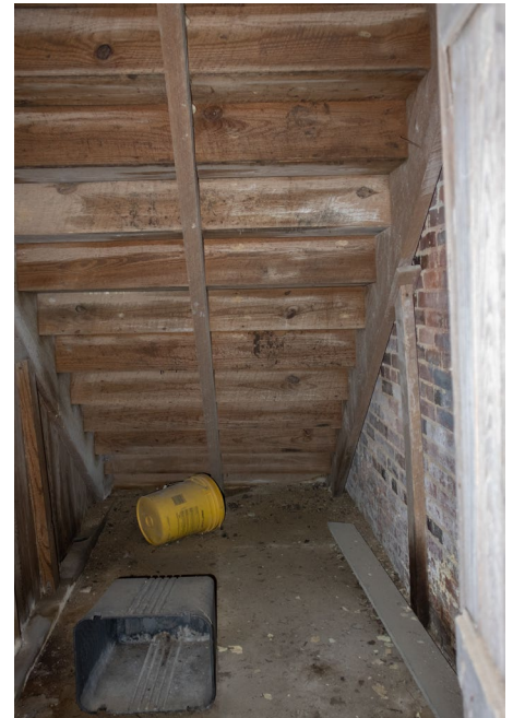
1C.12 Hallway – Interior of the small room under the stairs
