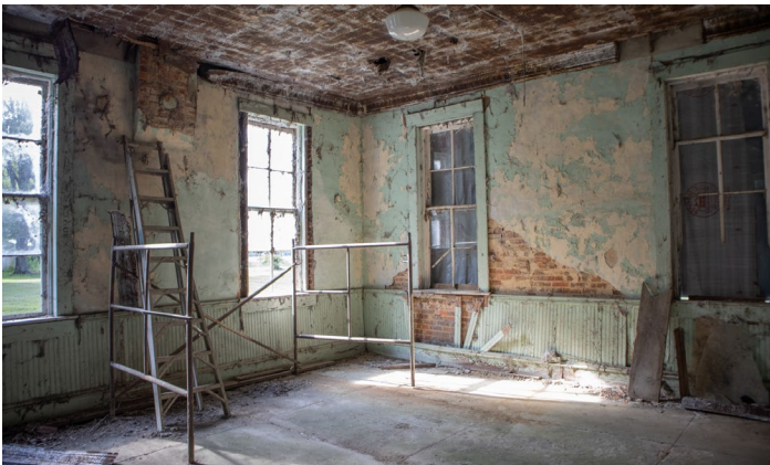
IC.21 Room A – Looking Southeast – Notice chimney connection
