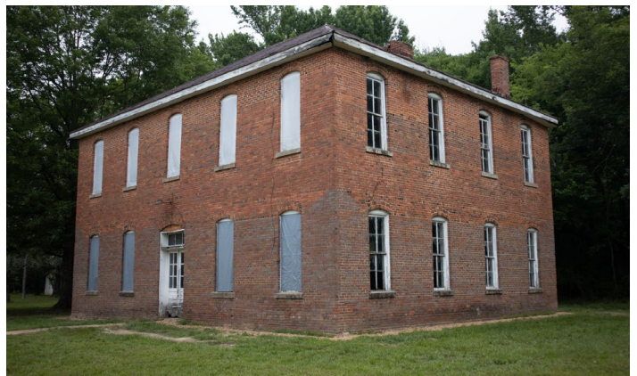
1A.6 Looking Northwest
