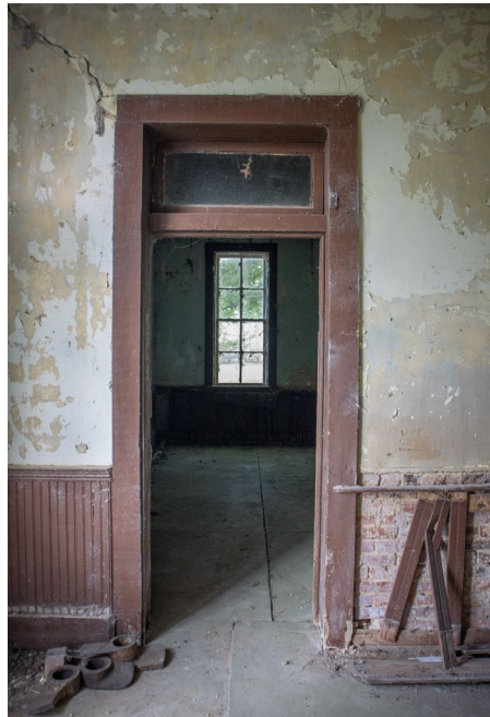
1C.17 Hallway – Opening looking into Room B – Door no longer remains
