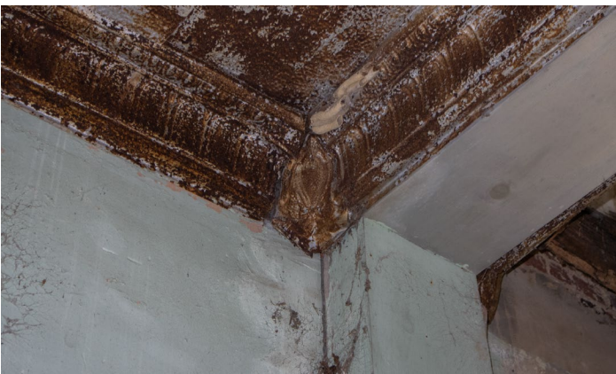
IC.29 Room A - Detail of pressed metal cornice corner
