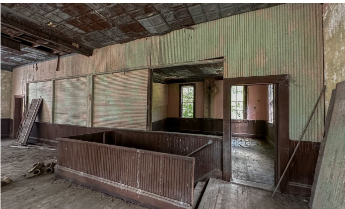
1D.5 Room A – Looking West into Room C
