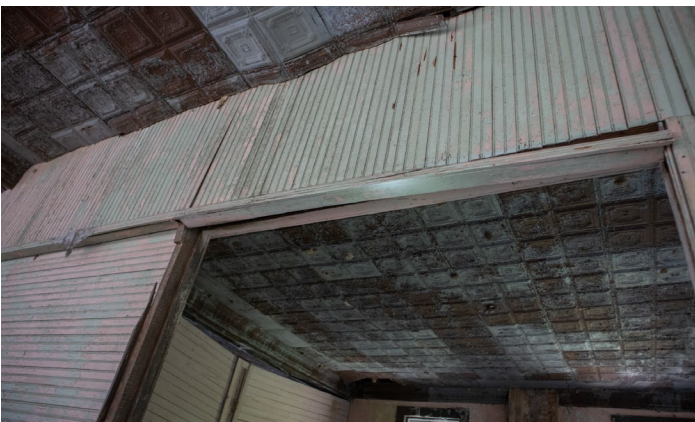
1D.26 Room C – Detail of counterweighted partition wall
