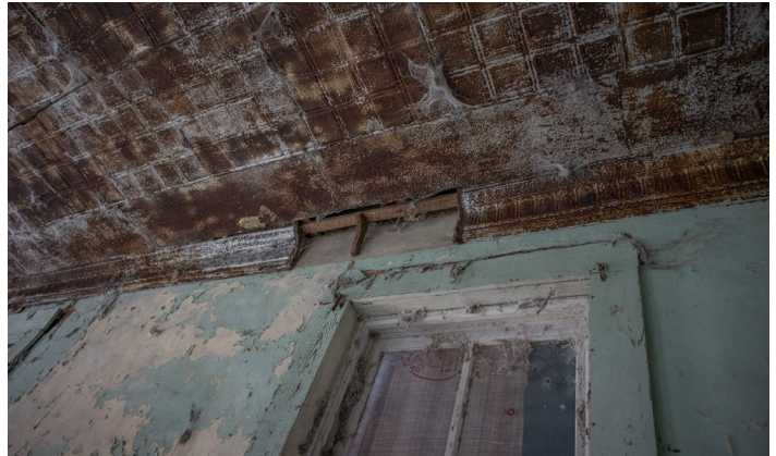
IC.28 Room A – Detail of pressed metal cornice
