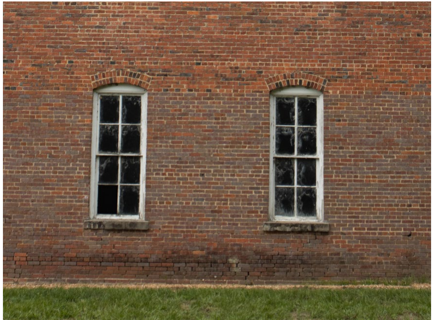
1B.27 East façade – Detail of the difference in brick coloration
