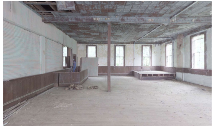
1D.8 Room A – Looking North
