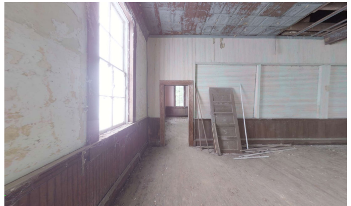
1D.9 Room A – Looking West into Room B
