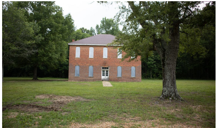
1A.4 Looking North - View of the building from the roadside entrance
