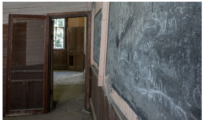
1D.21 Room B – Looking North into Room C – Notice a screened door
