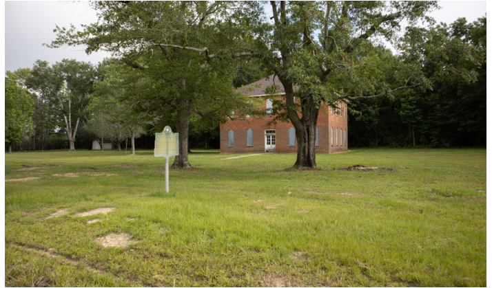
1A.2 Looking North - View of the building from MS-14
