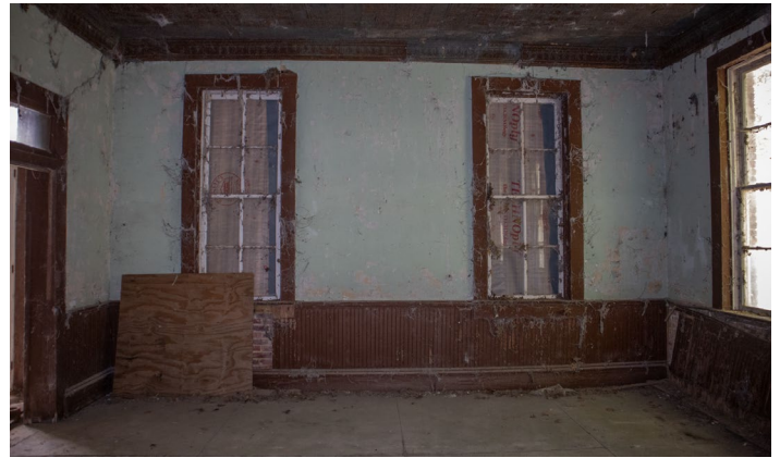
IC.36 Room B – Looking South
