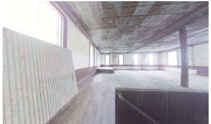
1D.4 Room A – Top of the Stairs looking East
