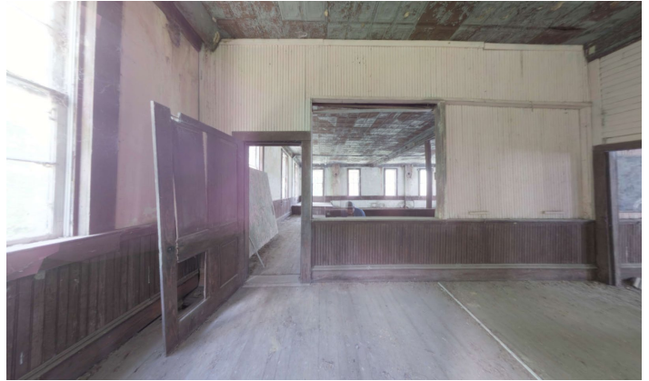
1D.23 Room C – Looking East – Notice counterweighted partition has been removed and placed at top of stairs
