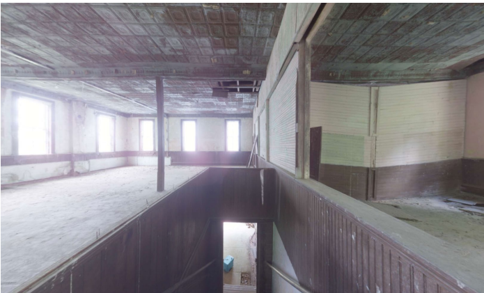
1D.3 Room A – Top of the stairs looking South
