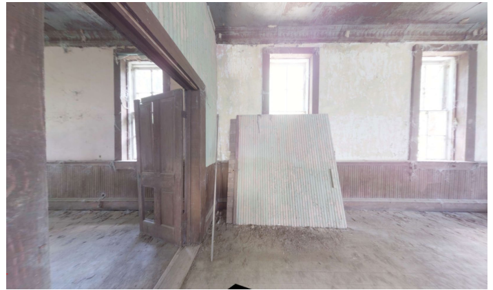
1D.2 Room A – Top of the stairs looking north
