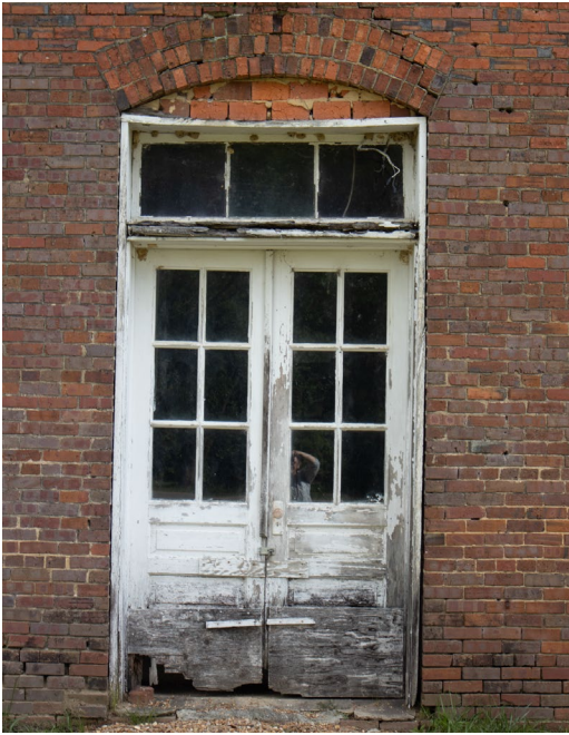
1B.1 South façade - Entrance door
