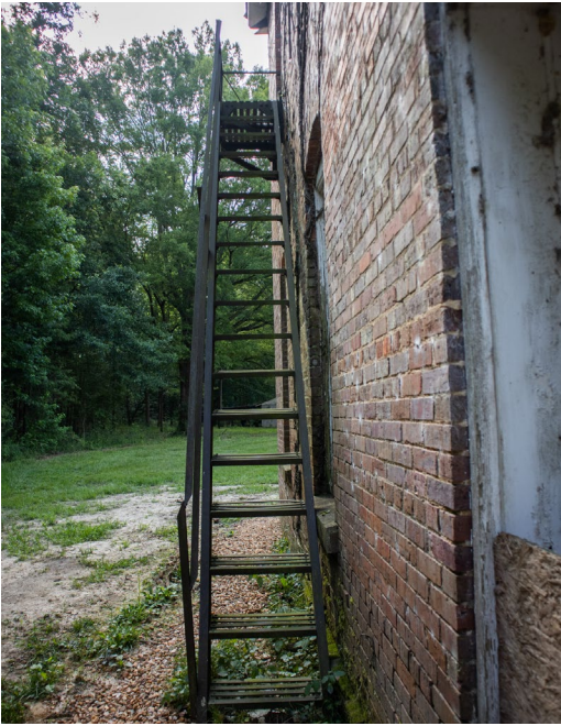
1B.16 North façade – Metal fire stair anchored into masonry exterior
