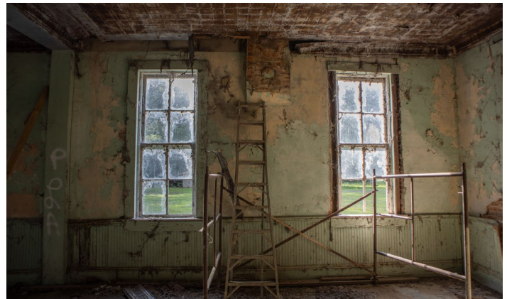
IC.22 Room A – Looking East – Notice chimney connection
