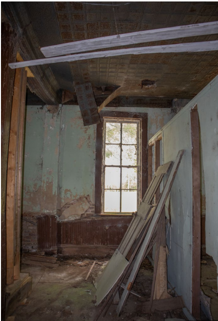
IC.48 Room B – Looking West
