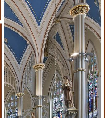
On the interior, an investigation of paint treatments, techniques and decorative elements were studied. Samples were created for approval. Intricate stenciling and design work in 23 kt gold leaf was implemented. Plaster was repaired and repainted, as well as Trompe l' oeil and other free-hand artistry.
