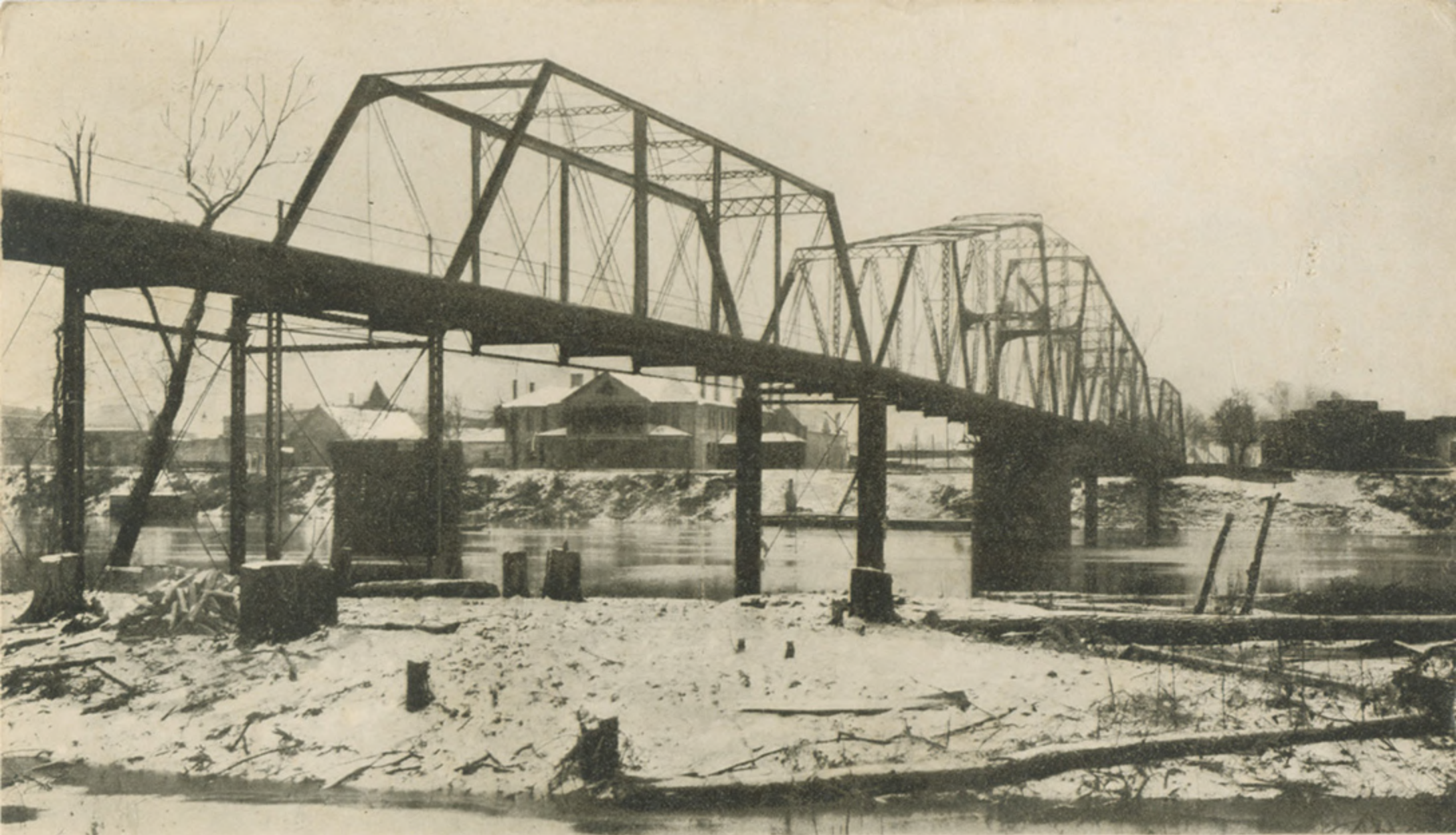
5784 The Bridge in Winter of 1895, Greenwood, Miss.
