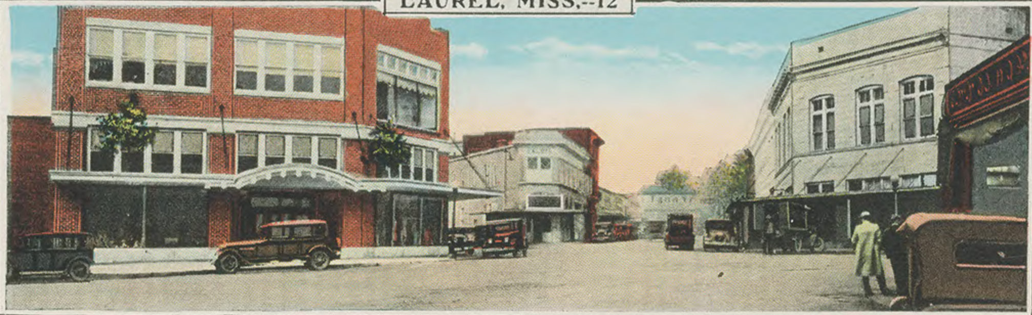
CENTRAL AVENUE LOOKING WEST FROM WOOLWORTH STORE
