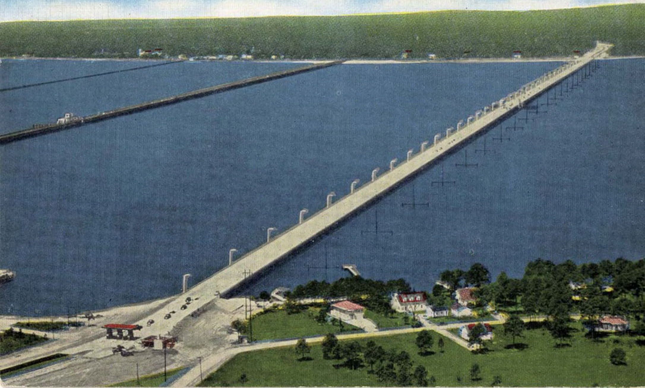
AERIAL VIEW OF NEW BAY ST. LOUIS BRIDGE, BAY ST. LOUIS, MISS.
