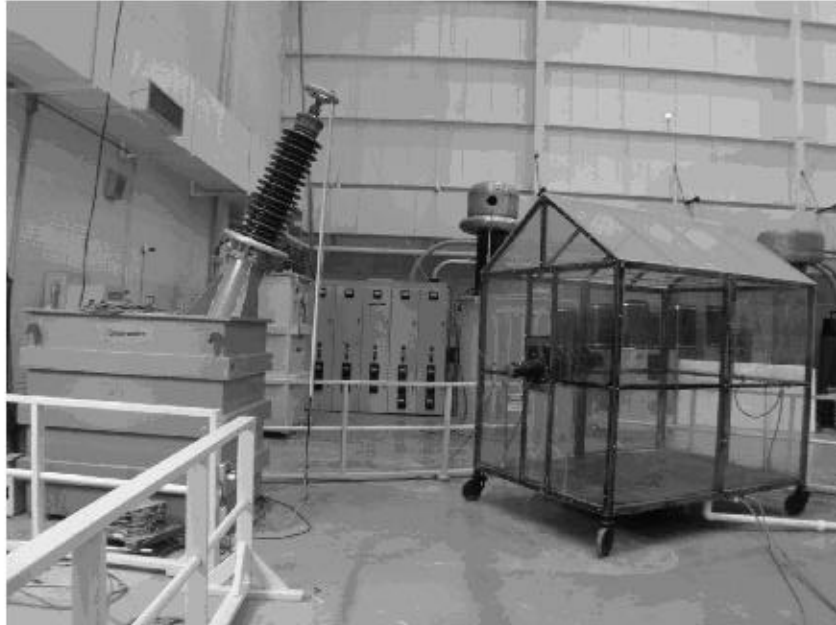
Fig. 4.1 The Setup of the Transformer and the Fog Chamber Used in the Accelerated Aging Tests.
