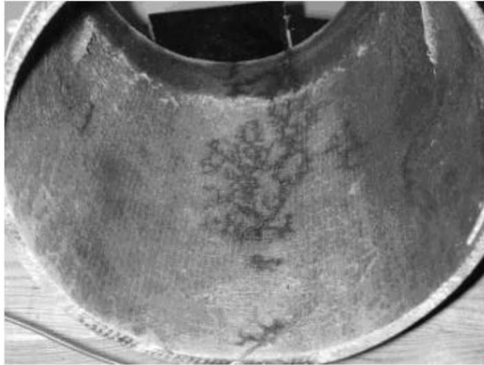
The Tracking Appeared on the Internal Surface of the Sample (No.4, With Some Scratches) After a 6 Hour Aging in Salt Fog Plus 25 kV/ft Electrical Stress.
