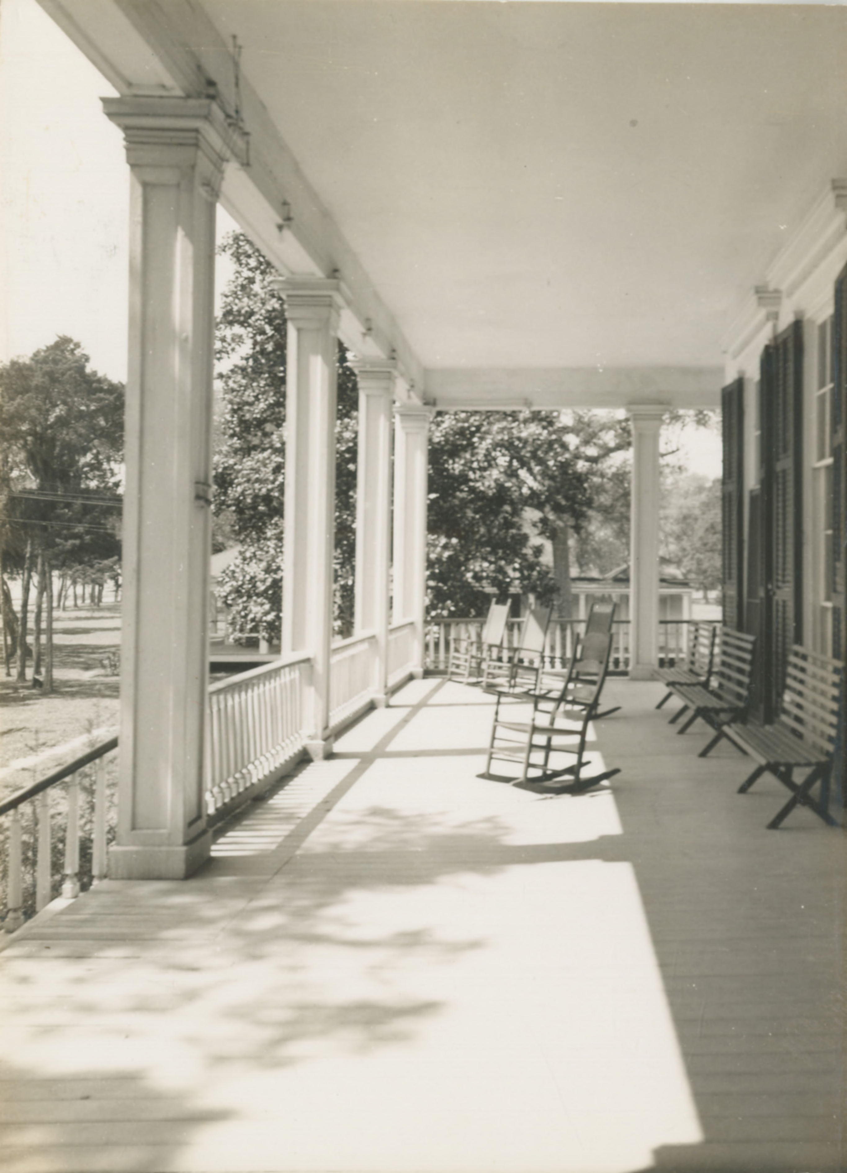
B-375 PORCH AND GALLERY AT "BEAUVOIR" - LAST HOME OF JEFFERSON DAVIS MIDWAY BETWEEN BILOXI AND GULFPORT, MISS.
