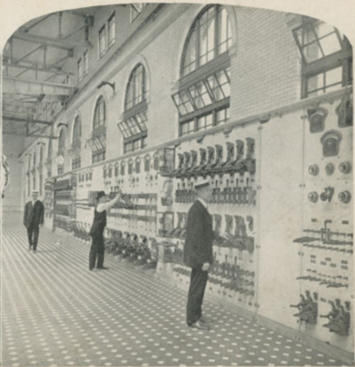
No. 40 THE GREAT SWITCHBOARD IN THE ENGINE ROOM. SEARS, ROEBUCK & CO., Chicago, Ill.
