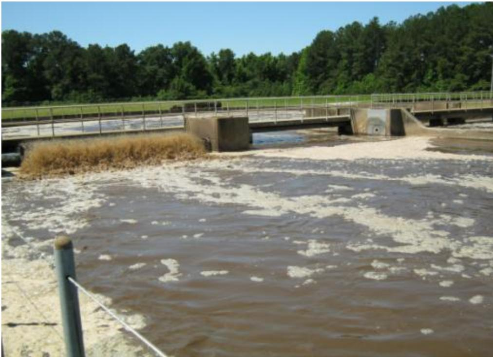
Figure B.2 Missing Aerator Assembly in Oxidation Ditch #2
