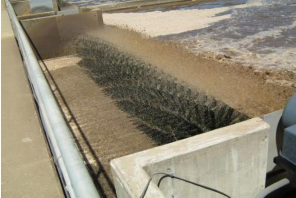
Figure B.1 Mammoth® Rotor Surface Aerator at Starkville WWTP
