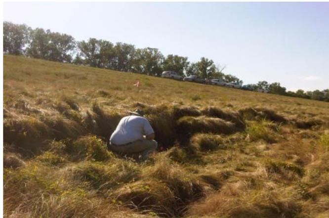
Figure 2.3 Typical levee slump slide
