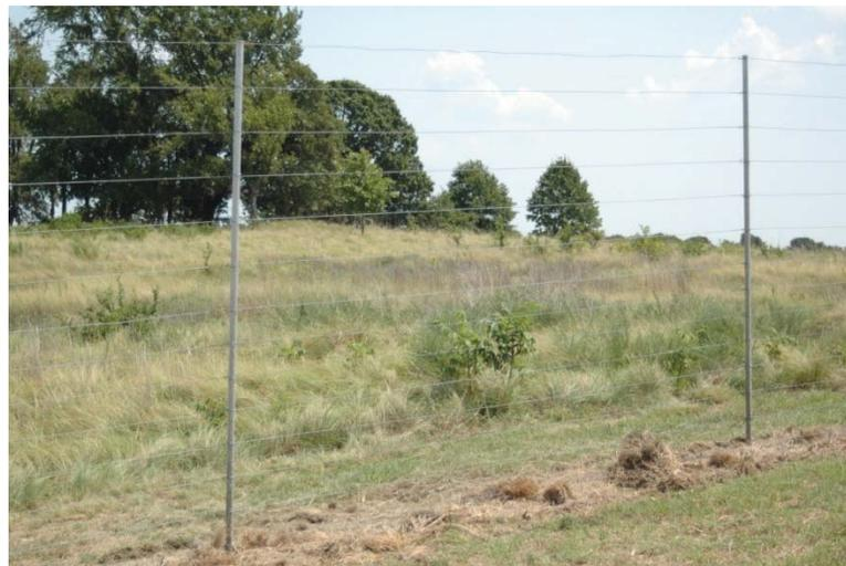
Figure 2.3 Photographs of the 15-strand high-tensile electric fence surrounding the Samuel Roberts Noble Foundation Wildlife Unit in Oklahoma. Height of fence was 2.5 m. Photos by Stephen L. Webb.
