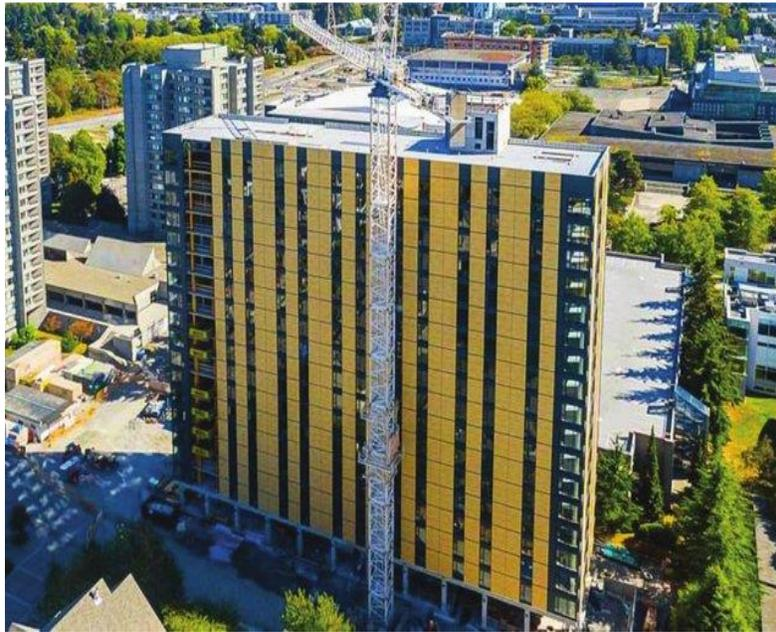
Figure 2.2 18-Story Tall wood Building (Hybrid Structure) built with CLT attached to glulam columns by steel connectors, located in Vancouver, Canada [6]
